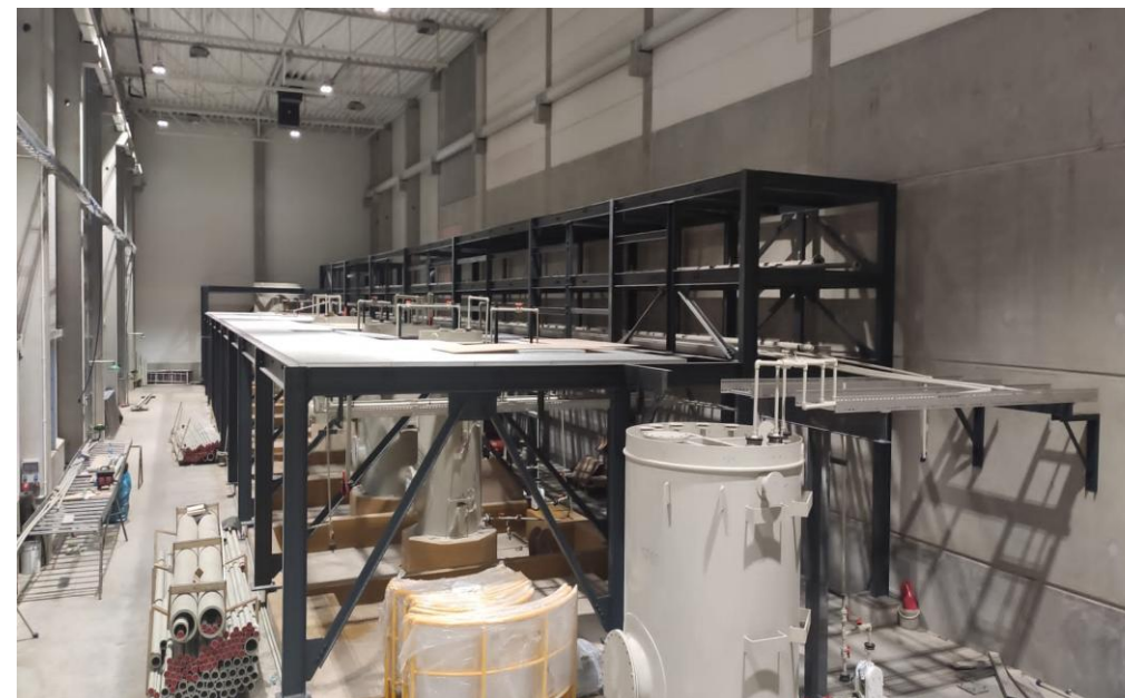
PHOTO FROM THE REALIZATION (ZERO MISTAKES DURING MANUFACTURING AND ASSEMBLY)
