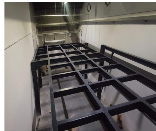
PHOTO FROM THE REALIZATION (ZERO MISTAKES DURING MANUFACTURING AND ASSEMBLY)
