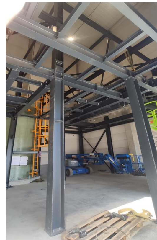
PHOTO FROM THE REALIZATION (ZERO MISTAKES DURING MANUFACTURING AND ASSEMBLY)
